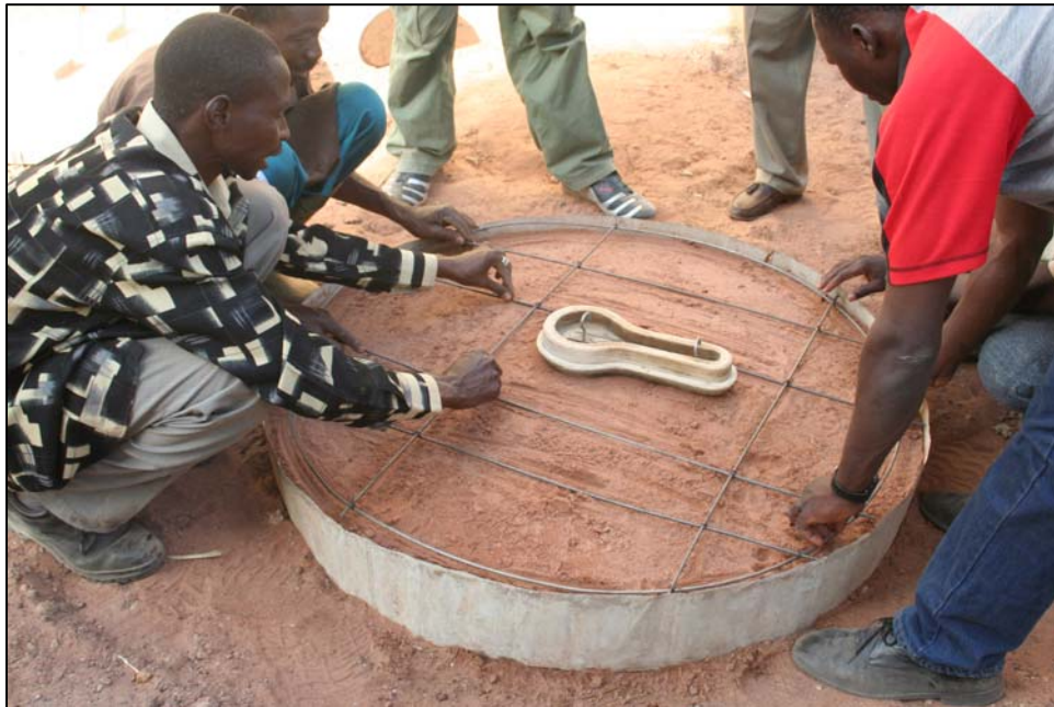
Masons in Mali prepare to pour cement into a latrine mold.
