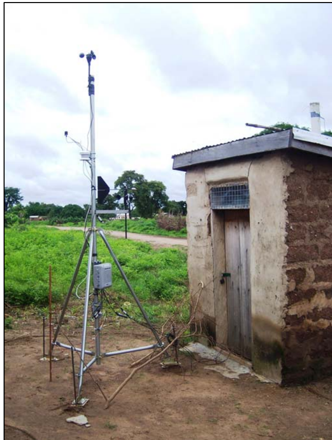
One of the VIP latrines studied in the Upper West Region of Ghana.
