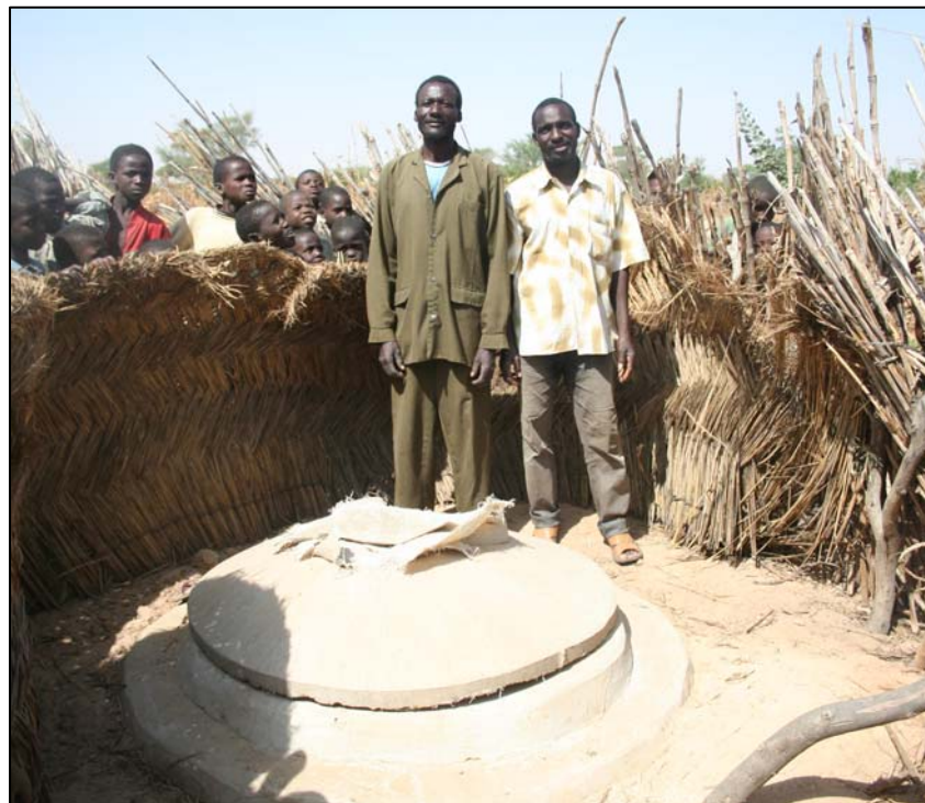
Community masons stand proudly next to a latrine with Sanplat slab.
