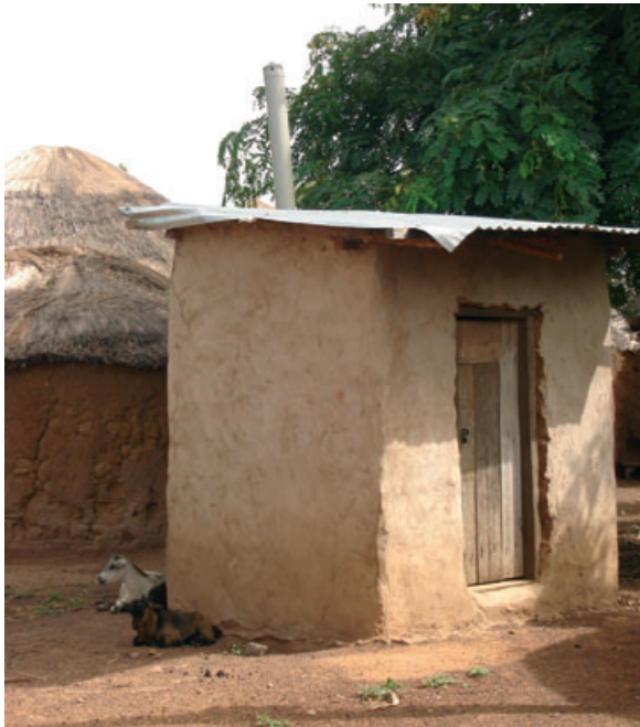
Figure 3 A completed ventilated pit latrine with a metal roof and plastered with cement is built to a higher standard than the owner's house made from mud blocks with a grass thatch roof.
